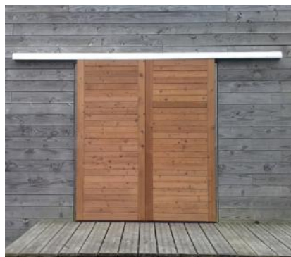
A LA POSE
