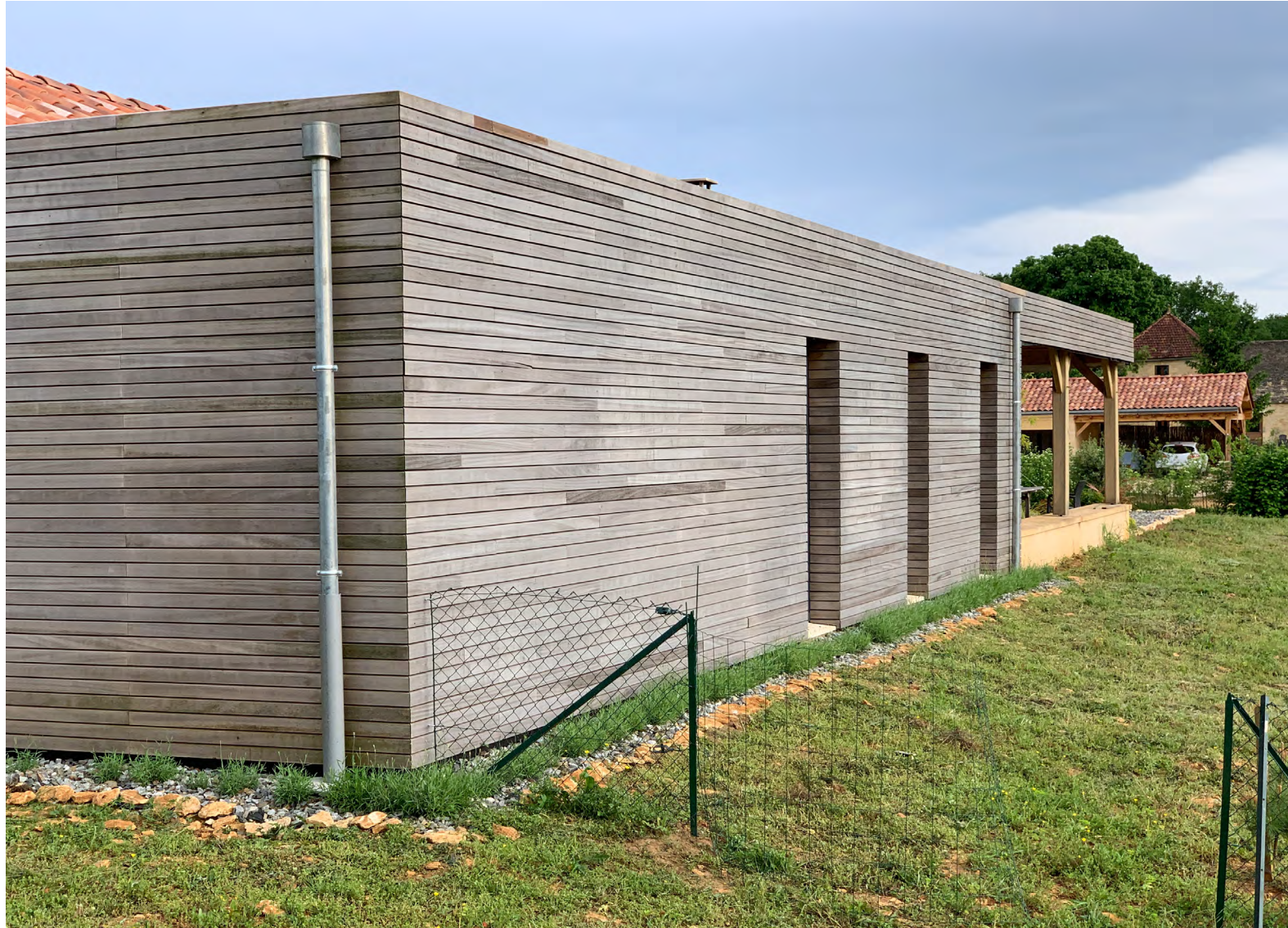
Project: Private House. Facade cladding in LDCwood® ThermoWood® ayous BELO profile. Planned by Lemahieu Group®.
