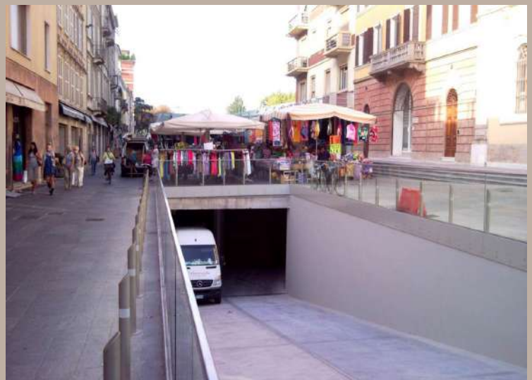
△ Before and after use of Top-Down NPS® solution for underground car park in Piazza Ghiaia in Parma.
