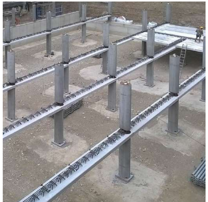
△ NPS® Cls beams supported on NPS® Slim columns allowed for the combination with hollow core slabs over 14 metres long.
