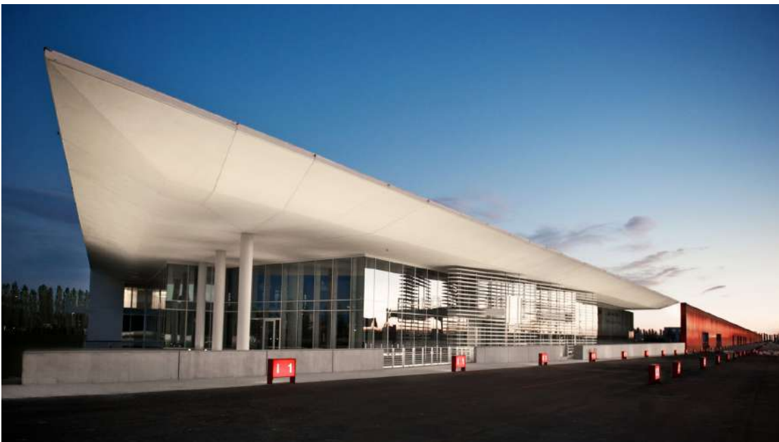
△ i.lab Italcementi, Bergamo – Architect Richard Meier.
