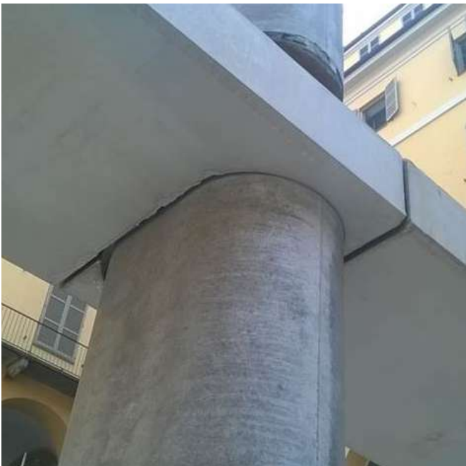
▽ NPS® Cls beam with shaped head surrounds the oval NPS® Style+ column.
