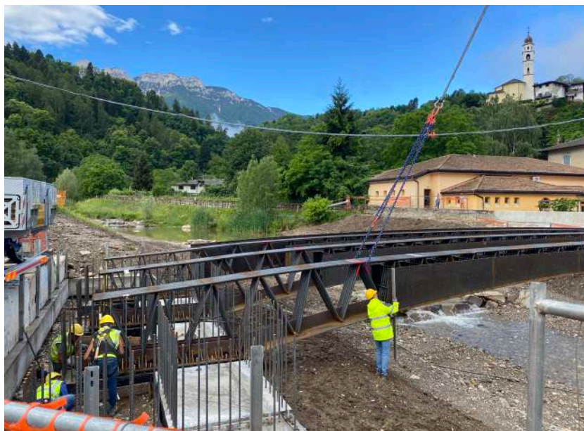
△ Construction of the single span bridge, Calceranica (TN).
