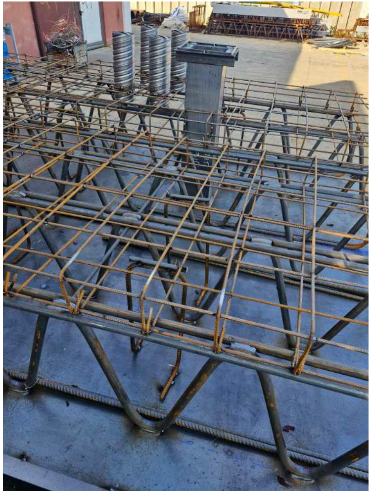
△ NPS® Strong slab for Megasider in Zaragoza.
