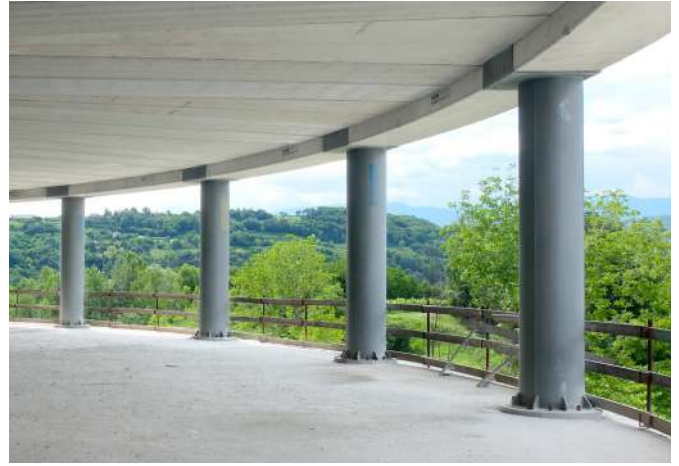
△ NPS® Cls curved beam, which adapts to the circular perimeter of the structure.
