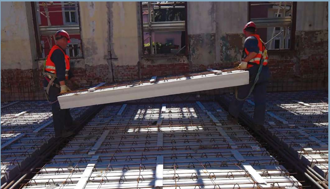
△ Thanks to its low self-weight Airfloor® allows easy handling on site.
